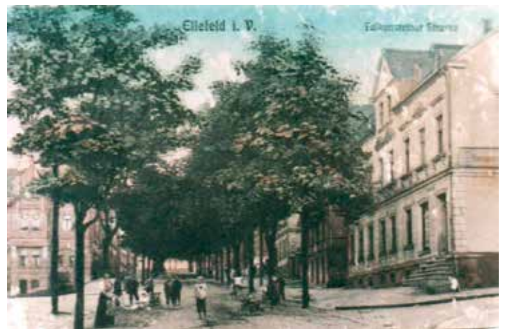
Blick in Falkensteiner Straße 1914
